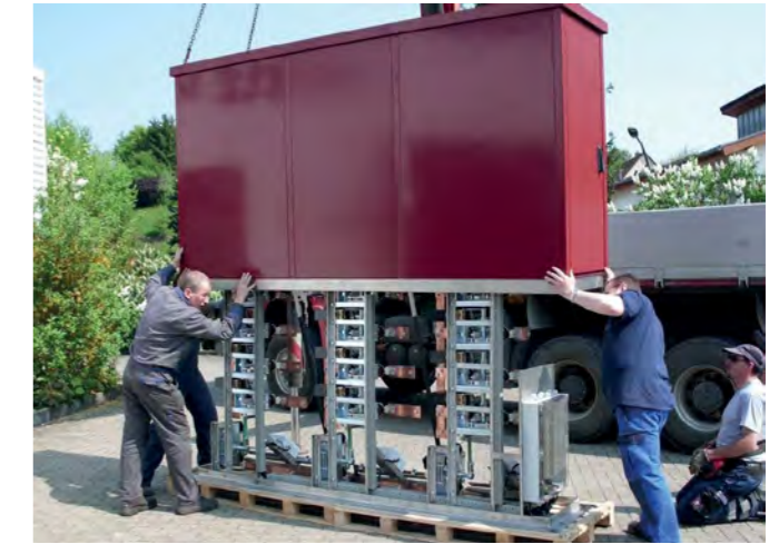
Cabinet housing railway control equipment.
